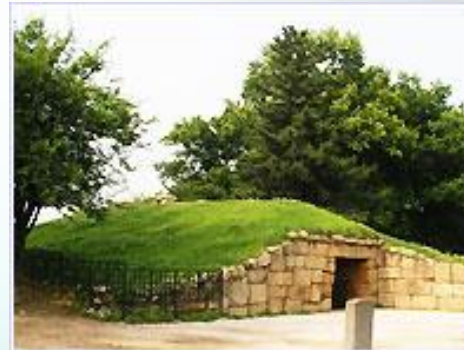
Ice Storage House
